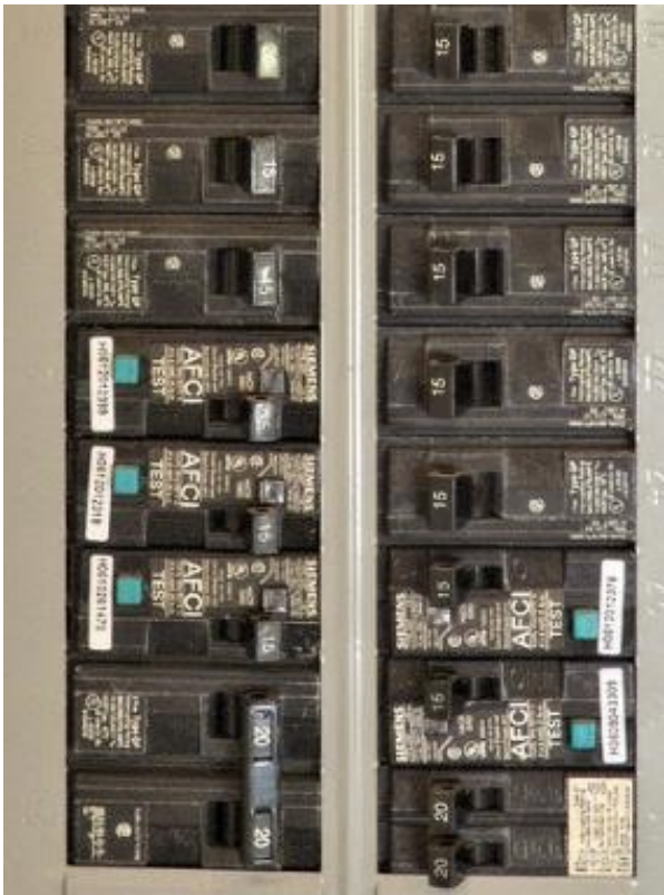
Figure 6. Breaker Box Equipped with GFI Breakers
